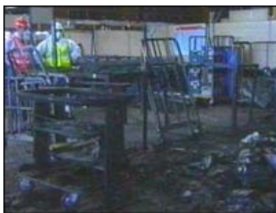
The grim aftermath of the sorting office fire
